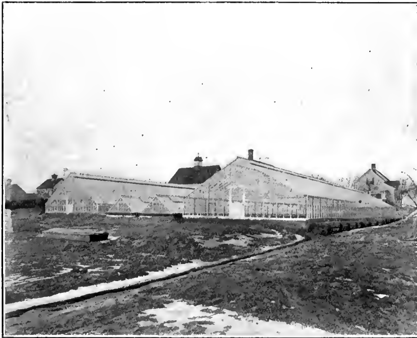
Houses of F. V. Metcalf in the great Ironqupit Vegetable Growing District, in which nearly 1½ miles of King Greenhouses were erected in 1907
